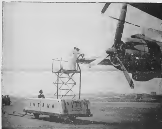
Intava, Company subsidiary for aviation business outside the United States, recently demonstrated at La Guardia Field a revolutionary new method of landing airplanes. The Intava "servitor" gets away from tank trucks, pumping gasoline with its own pumps direct from underground storage tanks to the airplanes. It also replaces landing, which can damage the landing gear and de-lasing equipment of a wing, with an "elevate" that lifts the returning crew to the level of the wing.
